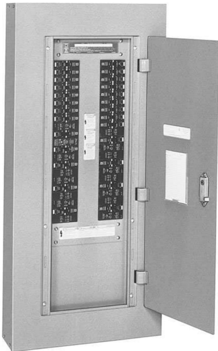
**9-5 Branch-circuit panelboard.** (Courtesy of Schneider Electric Company.)
